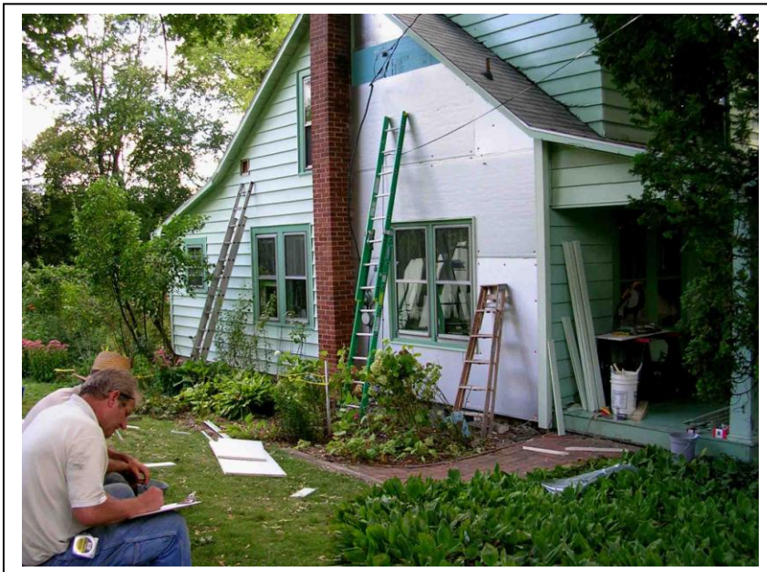
Right: Picture 3. East wall retrofit 2008, 2” foamboard over existing rock wool
