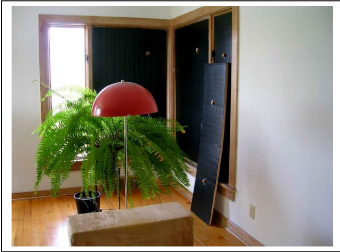
Above: Picture 1. Foamboard shutters in livingroom, 2000
