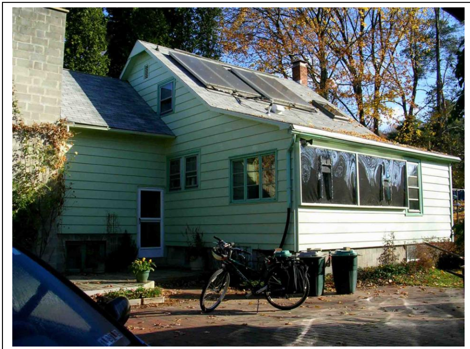
Above: Picture 8. Completed Kreamer hot air collectors, fall 2008
