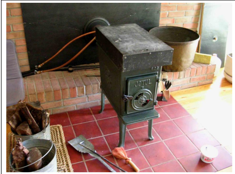
Above: Picture 7. Heat transfer box to move heat from stove to basement apartment via plumbing in Picture 6
