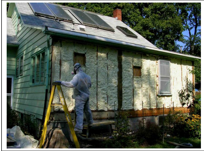
Left: Picture 4. Urethane foam being sprayed into stud cavities
