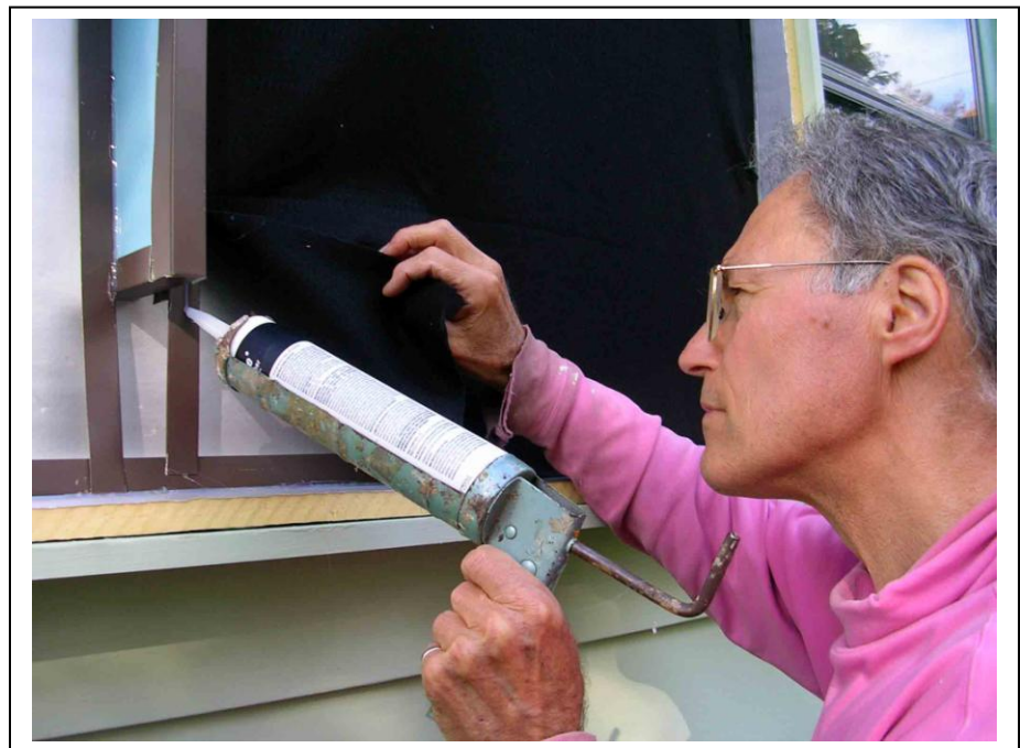
Right: Picture 7. Gene gluing black polyester felt using silicone adhesive
