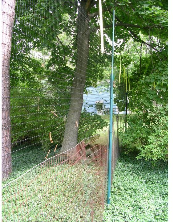
Here you can see more clearly the original welded wire fence with the taut black plastic deer netting spanning an additional three feet upward. The netting is secured with 20 gauge wire to a taut 14 gauge wire along the top edge and to the fence posts. It is also secured in spots to the fencing below it.
