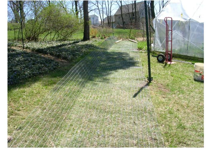
We use long 2x4's as a surface against which to bend the fence. You want 15" to 18" to run flat along the ground as a 1<sup>st</sup> level deterrent from burrowing critters. Don't bend to 90 degree angle. Keep it more shallow as shown so that weight of the fence will push it down to the ground once it is vertical.
