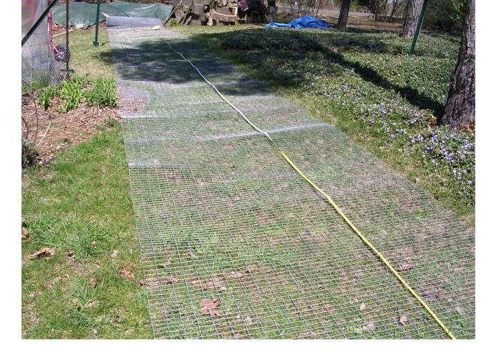
Here we have rolled out our welded wire mesh fencing which is 5 feet wide with 1" x 2" rectangular mesh – seems to keep the bunnies out pretty well though chipmunks get through. The tape measure runs along the 18-inch mark where we intend to bend the fencing. Date of this project was April 2007.
